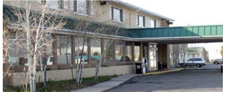
The Crossing, a Denver Rescue Mission facility.
